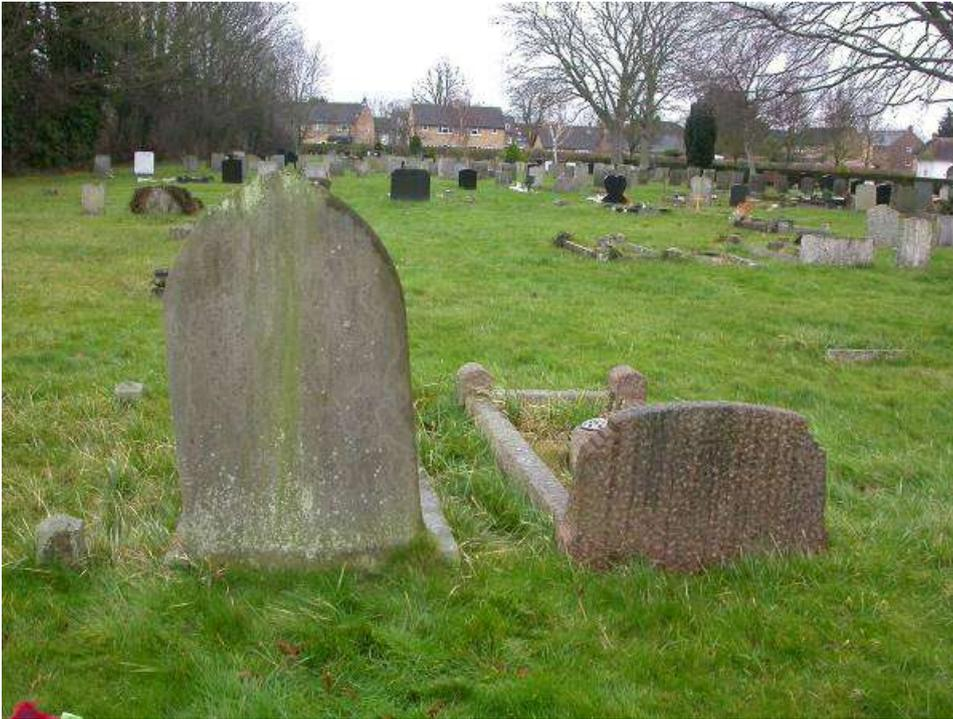
Fig. 13. A sandstone gravestone and a granite one. Being somewhat porous, the sandstone draws groundwater up by capillarity and this results in a 'tide-mark' indicating the upper edge of this zone, which is made more calcareous by lime in the ground water. The granite is impervious and shows no such phenomenon.
