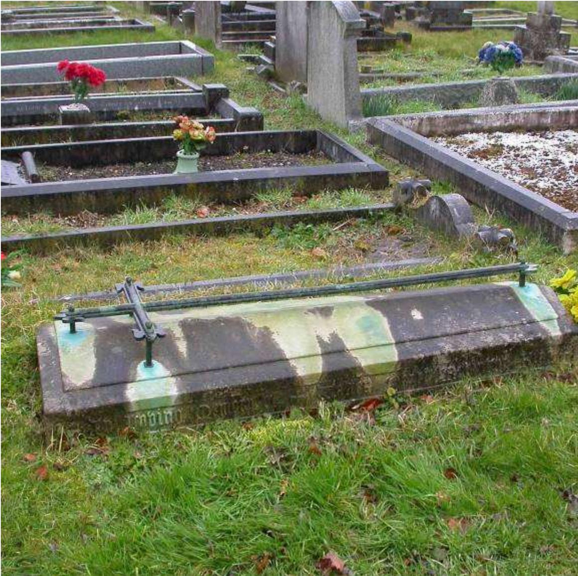
Fig. 12. A coped limestone tomb contaminated by copper run-off from a bronze cross. The most heavily contaminated rock is bare of lichens and is stained blue. Elsewhere the tomb is dominated by *Verrucaria obfuscans*, with small amounts of *V. nigrescens* and *V. ochrostoma*.
