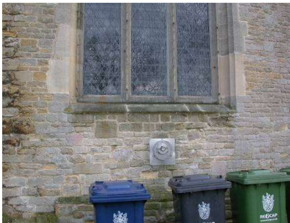
FIG. 11. Church buildings often support specialist metallophyte communities associated with various metal fittings. Here, the windowsill is dominated by Arthonia lapidicola which will have colonised when a former rusty window grille was present. Modern replacements, such as this galvanized grille, tend to be toxic to most lichens, though A. lapidicola is surviving here.
