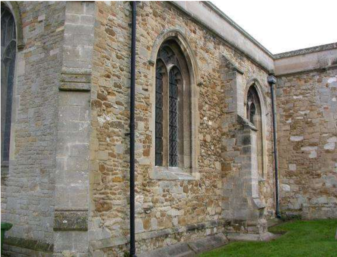
FIG 10. South wall of church, to west of porch.
